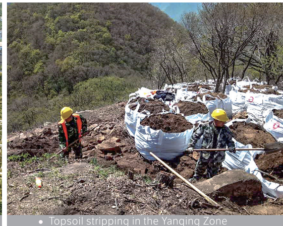
• Topsoil stripping in the Yanqing Zone
